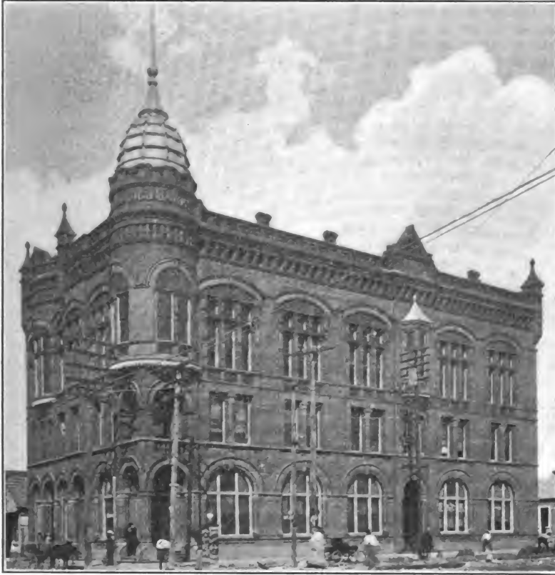
THE BANK'S BUILDING.
